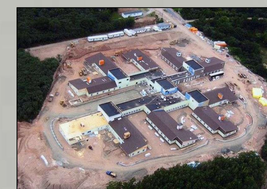
Construction Underway at Tideview Terrace, Digby Opening June, 2011
